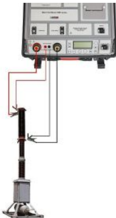
RMO-G cable connection on live tank circuit breaker
